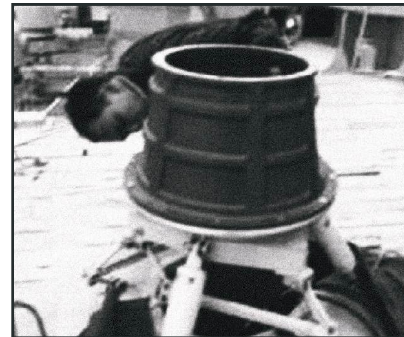
INSTALASI SKM EOT
